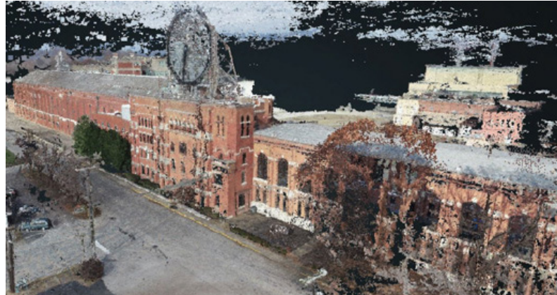
Point cloud from aerial survey of old Colgate factory
